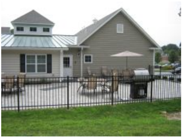
The Terrace at the new Chestnut Cottage
